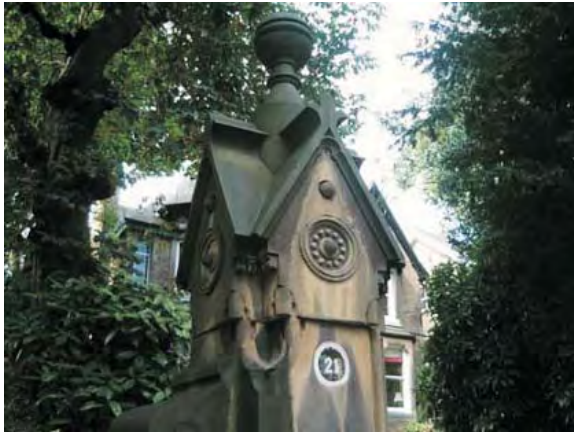
Ornate gate pier at No. 21 Southbourne Road
