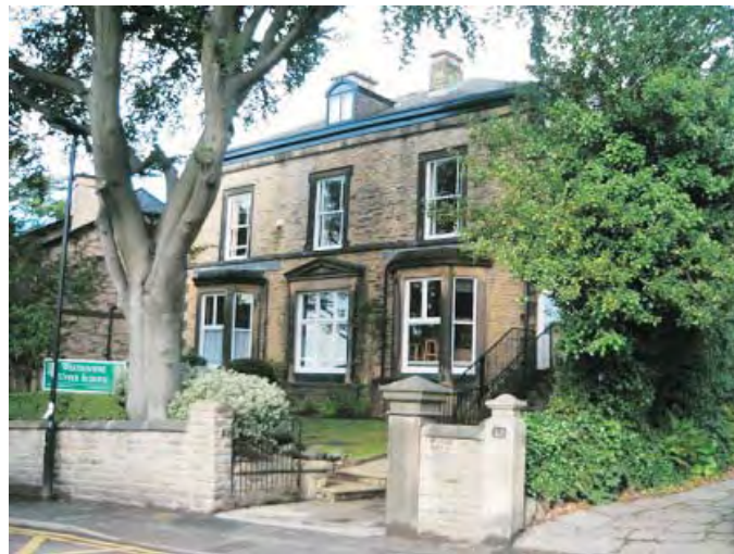
Nos. 50 and 52 Westbourne Road
