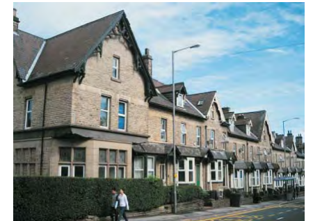
Nos. 116-126 Whitham Road (Dalkeith Terrace)
